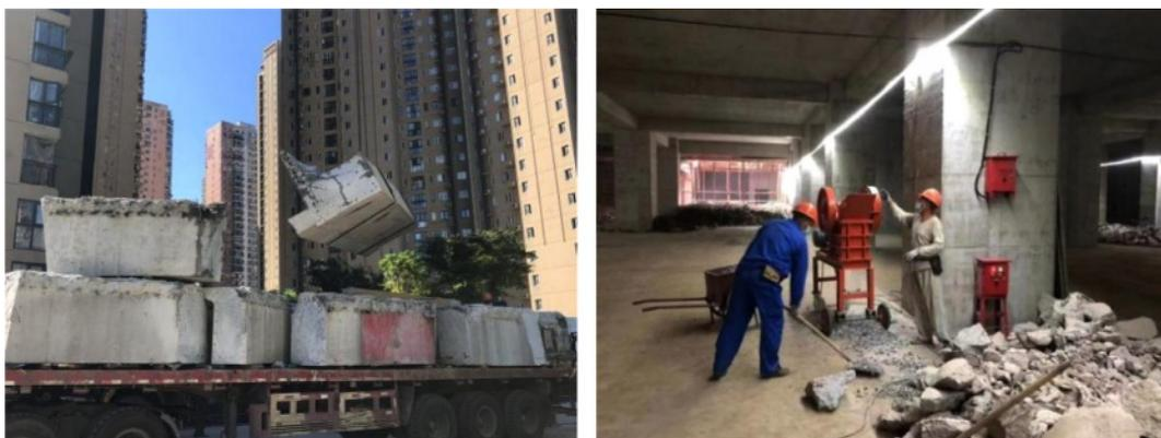
**Fig. 1.** Demolition of supported beams and crushing of waste cement.
