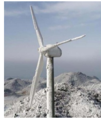
Fig. 1. Ice accretion on a wind turbine.
