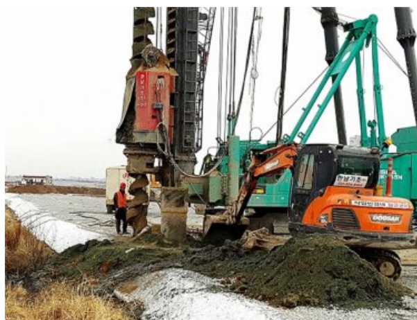
Fig. 1. Pile-supported embankment construction site.
