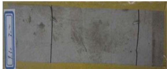
Fig. 1. Cracks formed on prismatic specimens by embedded method [13].
